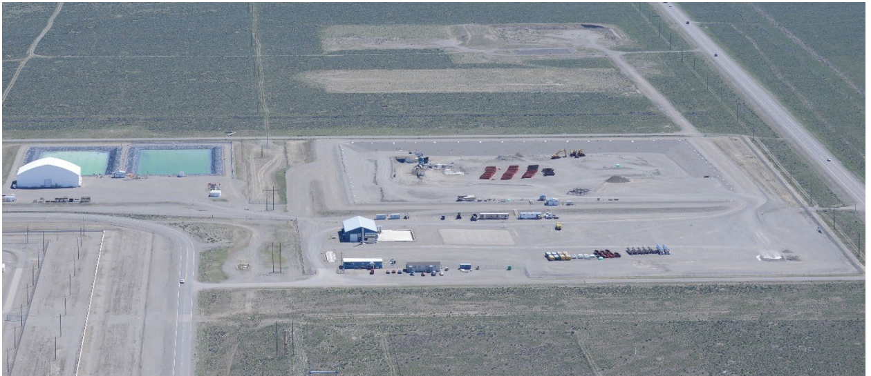
The Idaho Comprehensive Environmental Response, Compensation and Liability Act Disposal Facility is located near the Idaho Nuclear Technology and Engineering Center at the Idaho National Laboratory Site.
