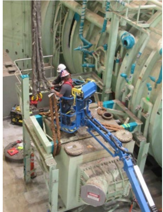
IEC crews remove a steam dump condenser from the westside of the S1W prototype.
